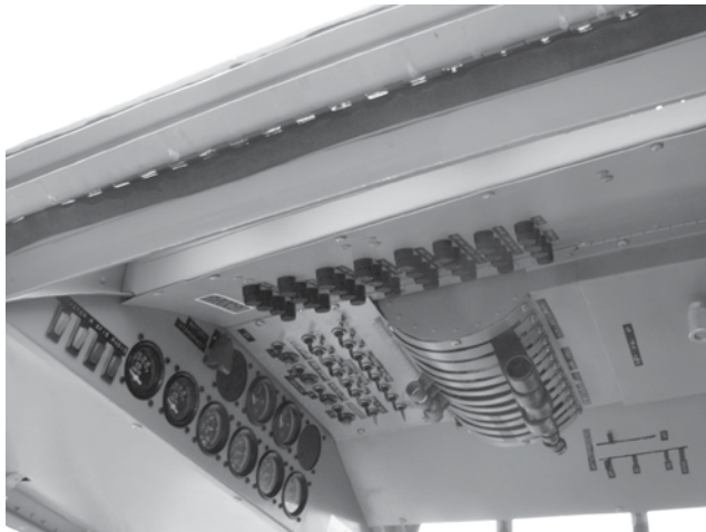
Top: Panel is a combination of electronics and steam gauges. Above, having four engines means four of every engine control and monitor.
